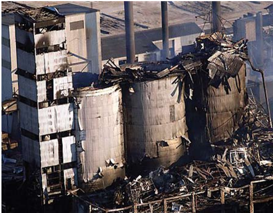
A massive combustibile dust explosion ripped through the Imperial Sugar Refinery in February.
